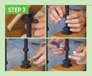
Once the baluster is installed, tighten and lock the baluster base, telescopic shaft and swivel top with the set screw. It is suggested to apply thread locking liquid on the set screws. Do not apply thread lock liquid on the swivel top until it is securely screwed into the handrail.
